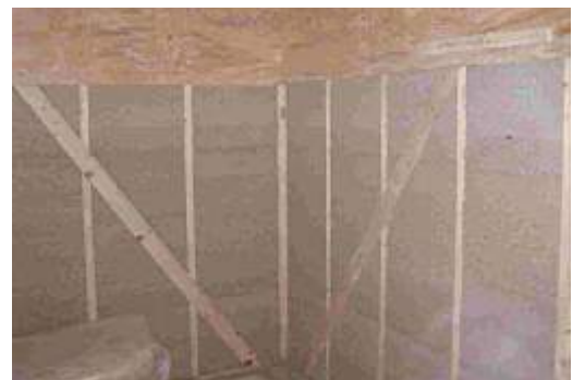
Figure 8: Infill of timber frame structure with hemp hurds and lime ( www.oldbuilders.com )
