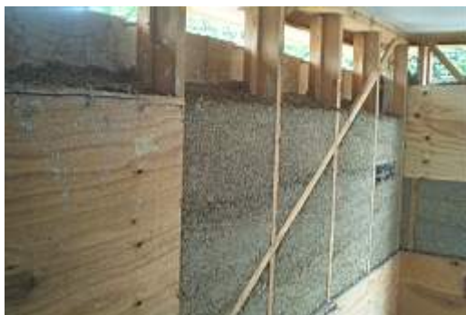
Figure 8: Infill of timber frame structure with hemp hurds and lime ( www.oldbuilders.com )
