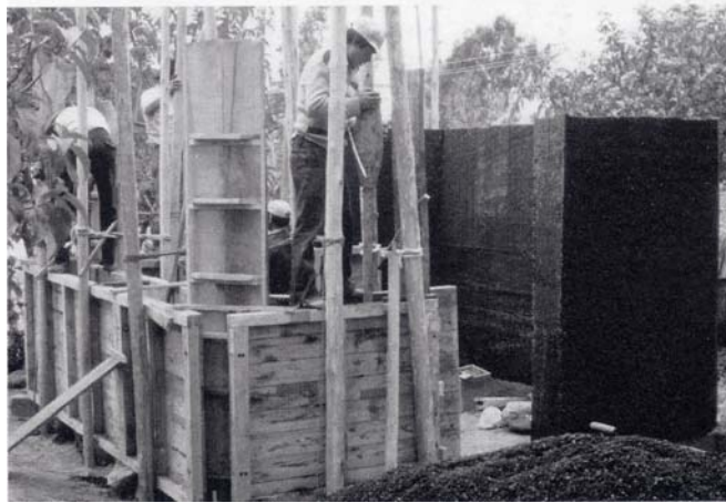
Figure 14: Light earth being placed in-situ (Minke 2000)
